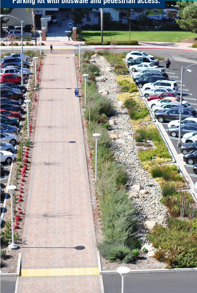
Parking lot with bioswale and pedestrian access.
