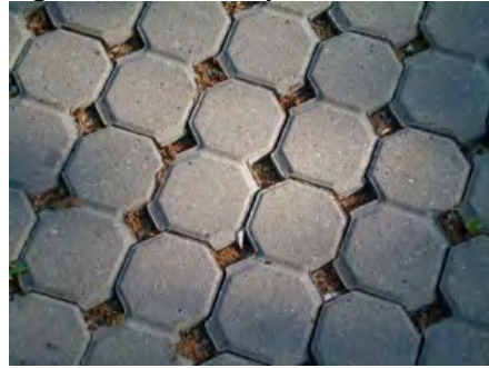
Figure 6: An Example of Porous Paving
