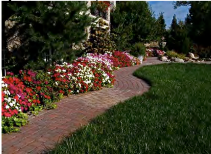
Figure 5: Permeable Clay Brick Pavements
