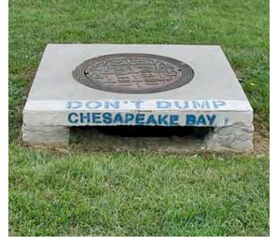
Figure 5: Storm drain marking
