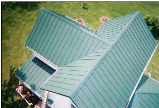
Figure 7: A Typical Residential Roof
