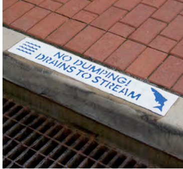
Figure 3: Storm drain marking
