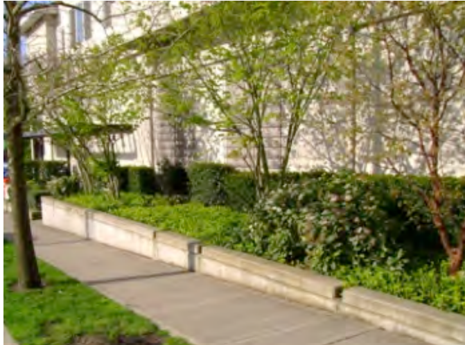
Figure 4: Example of Stormwater Planter
