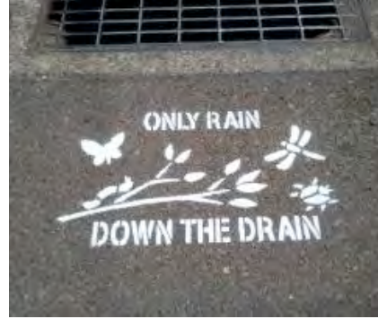
Figure 12: Spray Paint Marking
