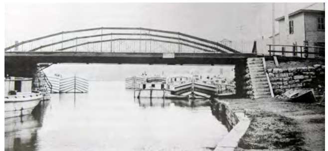
Figure 6: Whipple bridge over the Cayuga Seneca Canal
